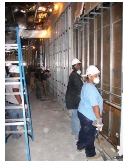
Reality House During (L to R): Dismantling studs, wiring, and wallboard. Loading out paper and cardboard. A NEW crew tackles a run of wall.
