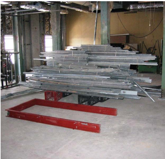
Figures 7,8: Reality House After. Studs and doorframes bundled for shipment. Paper, metals, and other materials prepped to go away. See Figure 2 for photo location.
