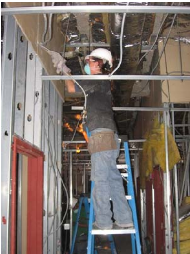
Figures 4, 5, 6: Reality House During. Dismantling studs, wiring, and wallboard. Loading out paper and cardboard. A NEW crew tackles a run of wall.
