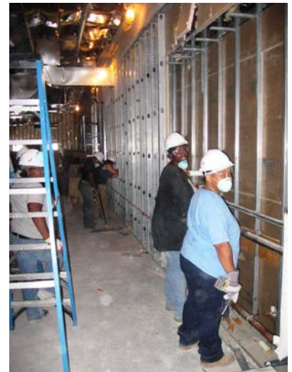
Figures 4, 5, 6: Reality House During. Dismantling studs, wiring, and wallboard. Loading out paper and cardboard. A NEW crew tackles a run of wall.
