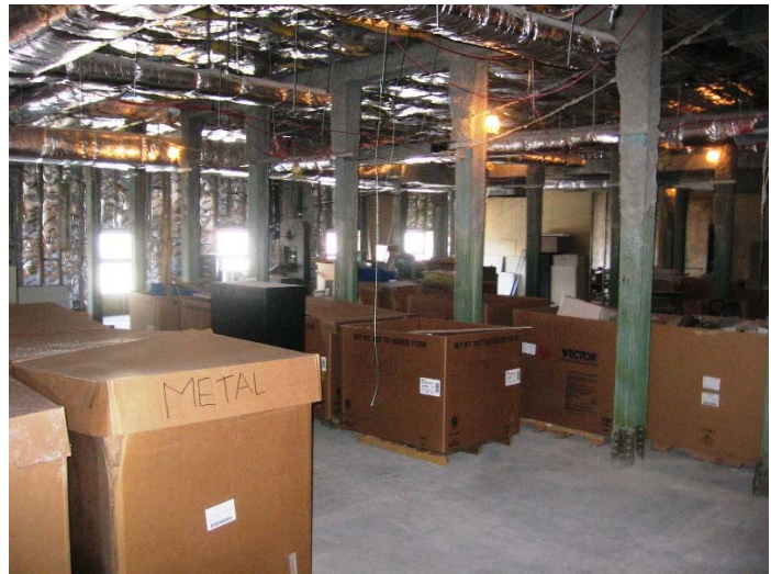
Figures 7,8: Reality House After. Studs and doorframes bundled for shipment. Paper, metals, and other materials prepped to go away. See Figure 2 for photo location.
