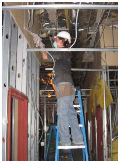
Reality House During (L to R): Dismantling studs, wiring, and wallboard. Loading out paper and cardboard. A NEW crew tackles a run of wall.
